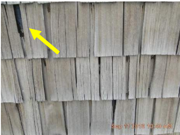
Large hole in shingles shows exposed ice and water shield below interlacing felt.
