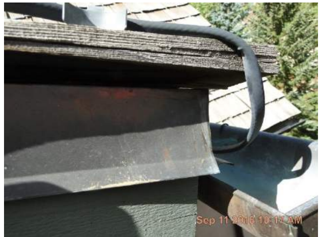
Close up of copper rake edge metal.
