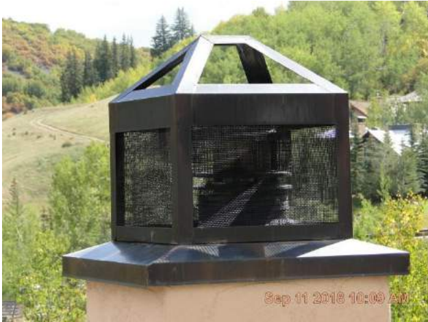
Copper chimney chase with screened cage around chimney flue. Chase is riveted and soldered together.
