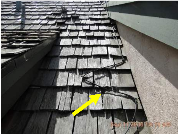
Side wall right of the front dormer shed roof with heat tape installed.
