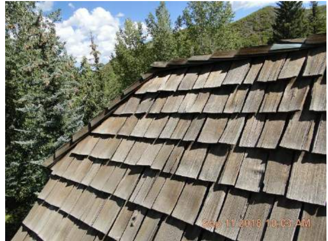
Left (west) slope of rear dormer.
