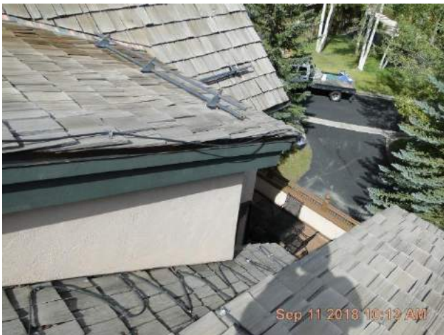
Front side wall view from top of roof shows fascia at gables, heat tape and side wall.
