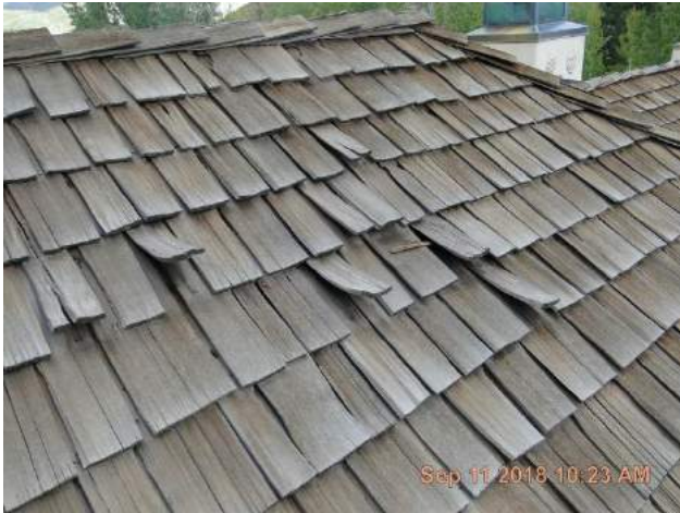
Badly curled wood shake shingle at the back roof slope.
