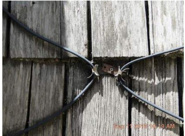
Heat tape is attached with copper clips.
