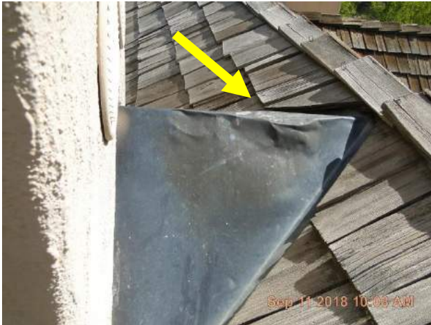
Damaged saddle / cricket.
