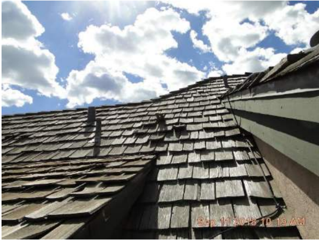
Wood shake shingles at front roof slope.
