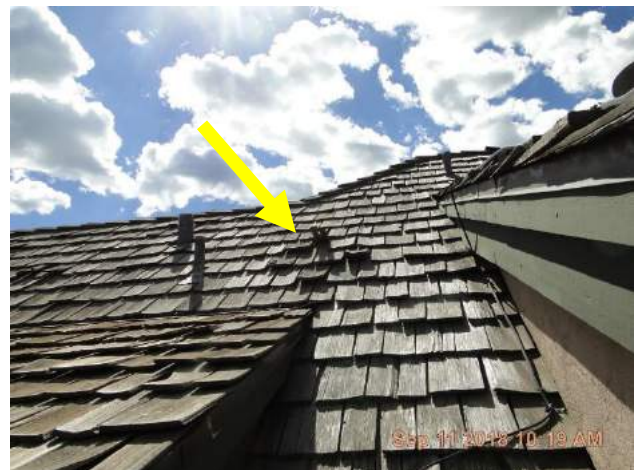
Back roof slope shows curled shake shingles.
