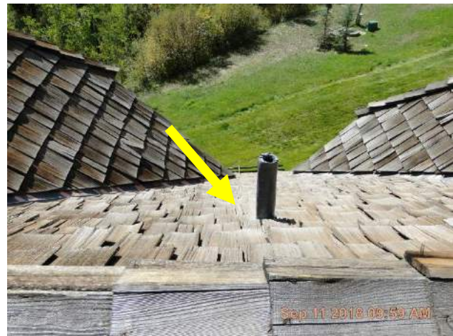
Roof slope at back elevation from top of roof shows lead pipe jack.
