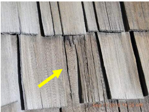
Badly split wood shake on back slope.
