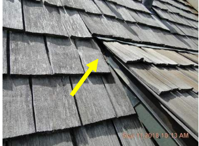
Front slope side wall at lower slope dormer. Shows The side wall flashing and rake edge metal.
