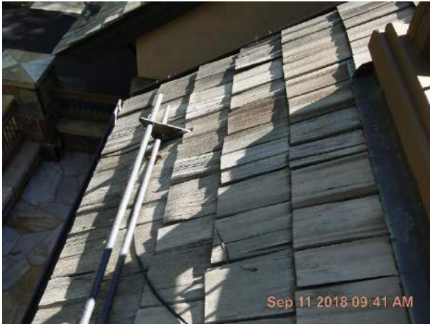
Front lower roof below deck shows head wall flashing and snow fence.
