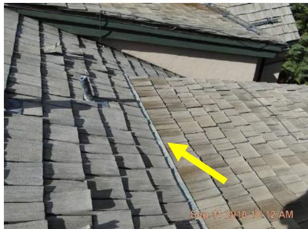
Transition from steep 7.5 slope roof to 2.8 slope roof.
