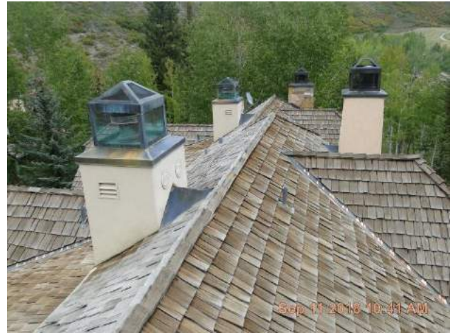
Top of roof from the west end facing east.
