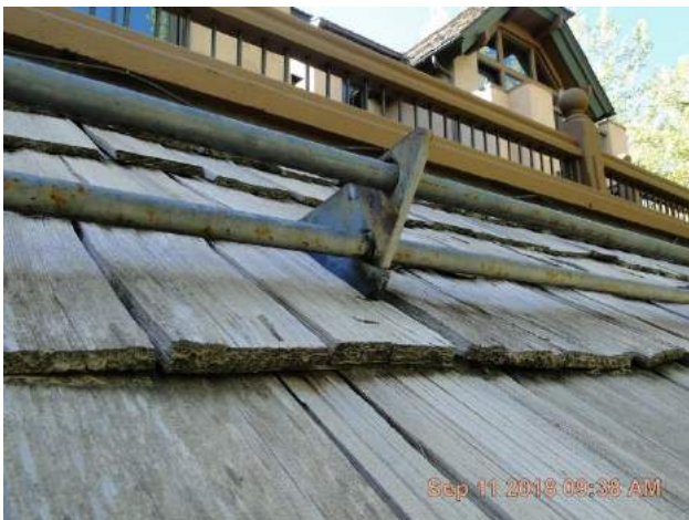
Snow fence at the front lower roof.
