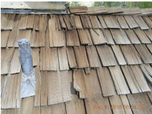
Split and worn wood shake at the back (south) slope. Wood shake shingles on the back slope are significantly thinner than the front slope due to weathering.
