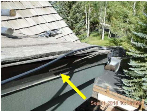
Rake edge metal at front dormer shed roof.
