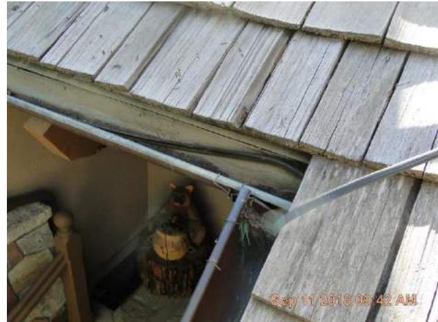
Front eave over entrance.
