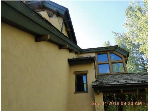
Front (north) elevation right side.
