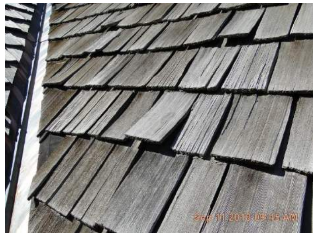
Left (east) slope of large front dormer roof to the right of the front entrance.
