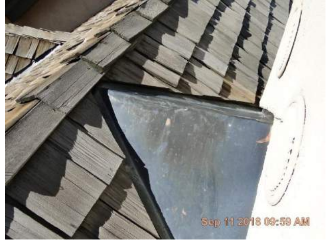
Close up of copper saddle / cricket.
