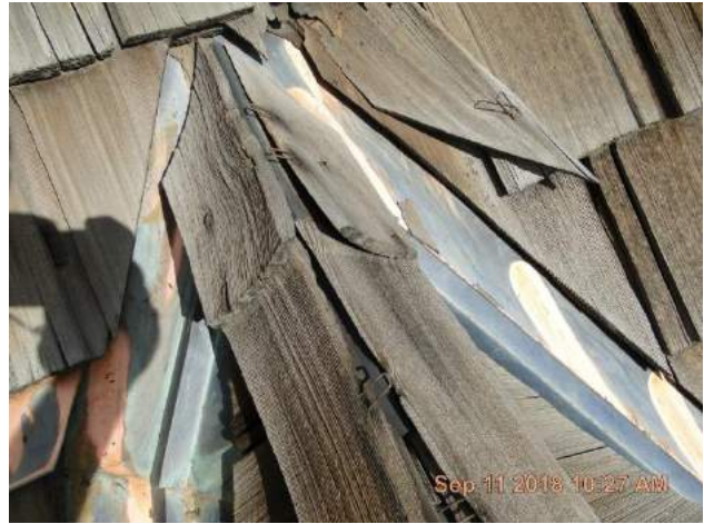
Ridge cap at back slope is split from the 2-inch staples rusting out. There is 10-inch copper step flashing installed under the wood shake at the ridge cap to protect the roof.
