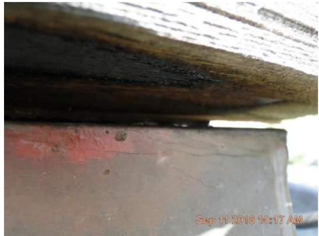
Close up of copper drip edge and wood shake starter.
