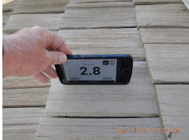
There are several lower slope dormer shed roofs that register at a roof slope of 2.5 to 3 requiring double felt.
