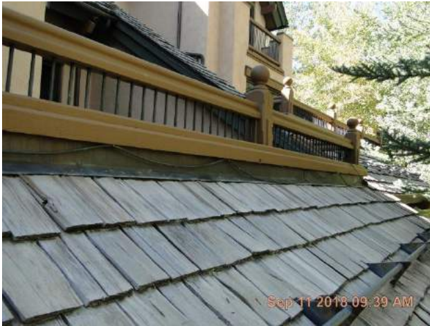
Deck with head wall flashing at the front lower roof.
