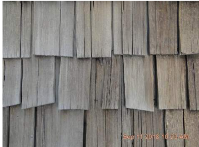
Weathered and split wood shake at the back slope.
