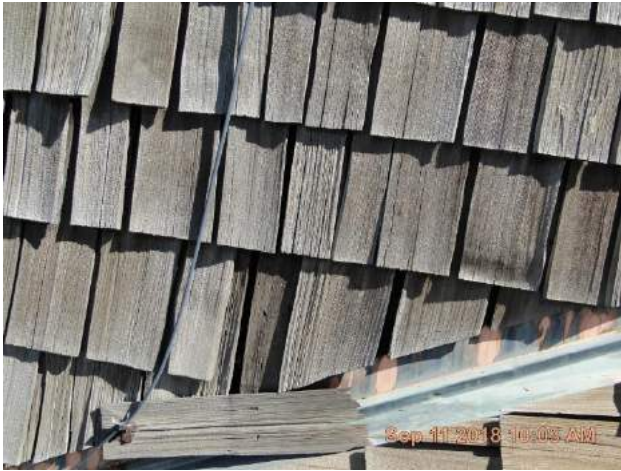
Wood shake at front dormer has detached.
