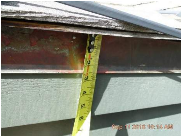
Copper drip edge metal is 2.5" high at the eaves.
