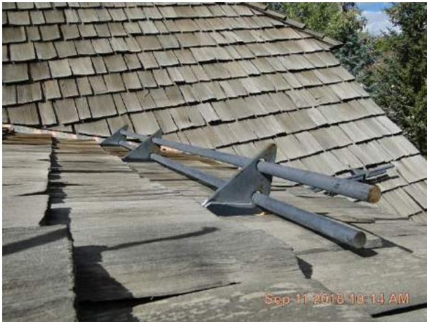
Snow fence installed on front dormer shed roof.
