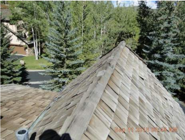
Front steep slope dormer facing northeast
