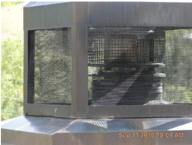
Closeup of copper screened cage at chimney flue.
