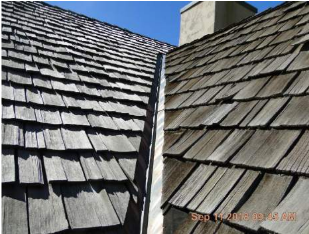
Copper W-valley at front slope where it meets the large dormer at the right (northwest) side.
