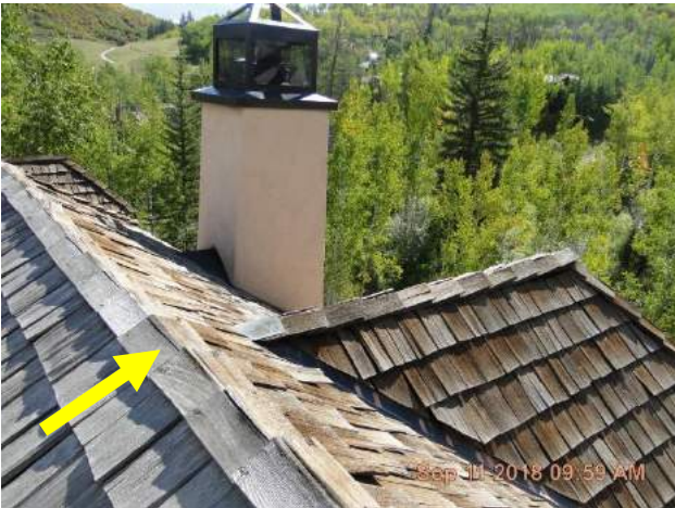
Top of roof facing south shows ridge cap.
