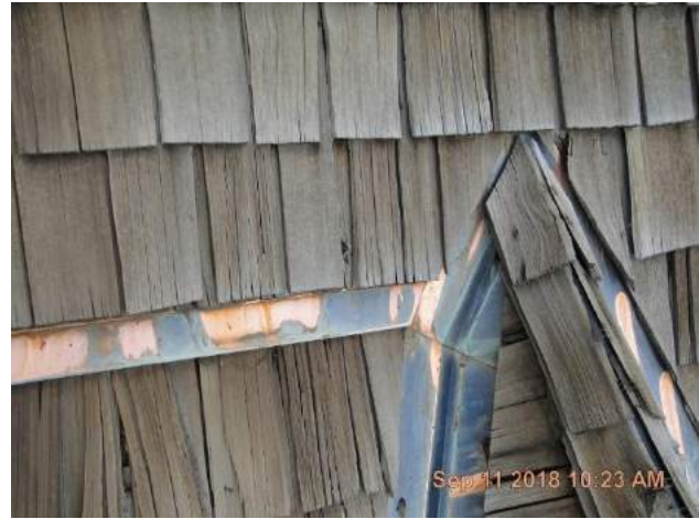
Copper transition metal and W-Valley metal at back, rear dormer
