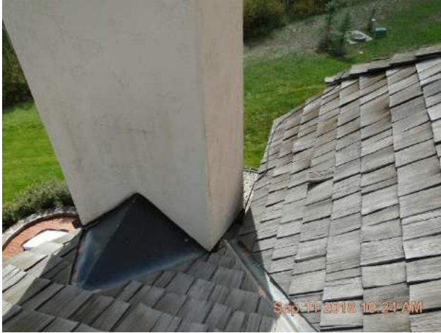
Chimney with copper saddle / cricket. Valley dead ends at the chimney side wall.
