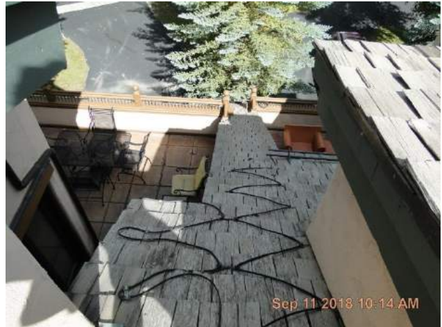
Front roof slope between decks shows heat tape.
