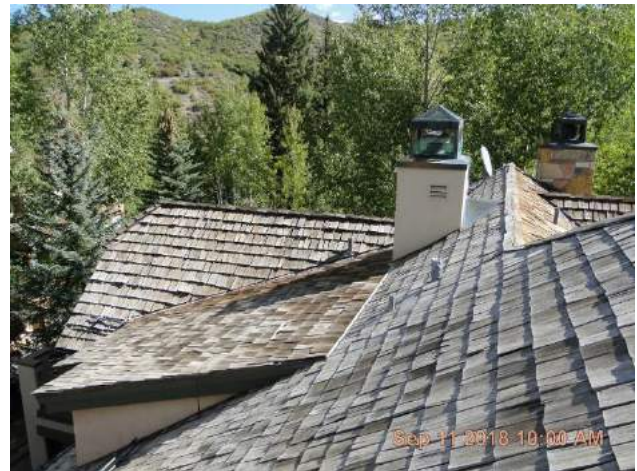
Top of roof from the middle facing east.
