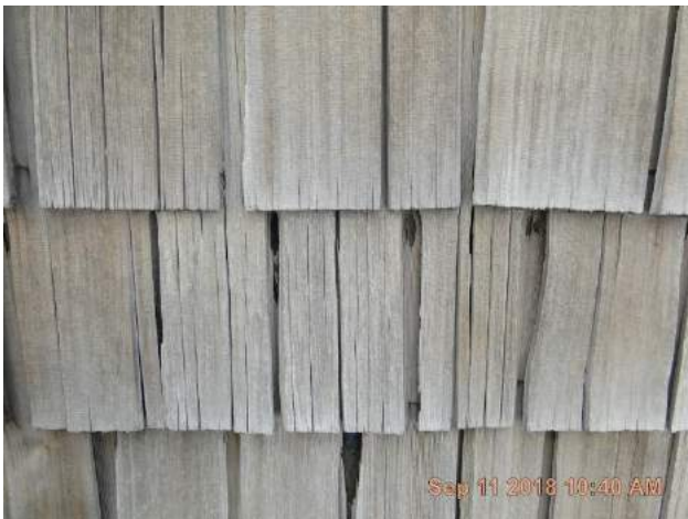
One section at the back slope shows weathered and split wood shake with 4 holes worn through them.
