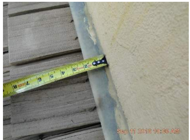
Head wall flashing is only 2-inches wide
