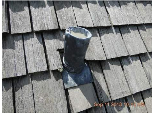
Close up of lead pipe jack.
