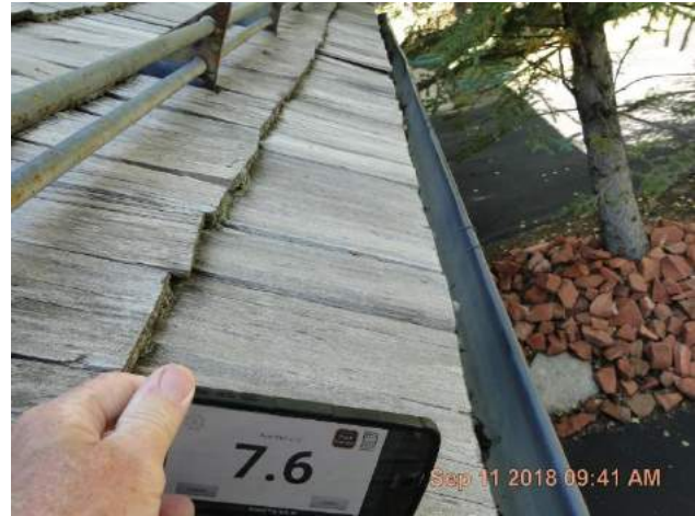
Roof slope reads at 7.5 in 12 slope which is a steep slope roof.
