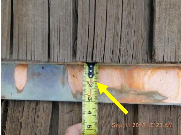
Copper transition metal is only 3-inches wide.
