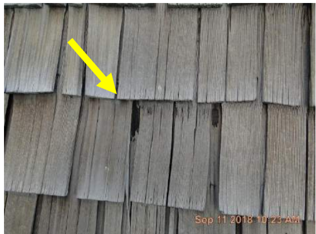
There are a significant number of wood shake shingles on the back slope with holes in them.
