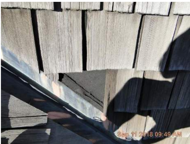
Close up shows missing shake shingle.
