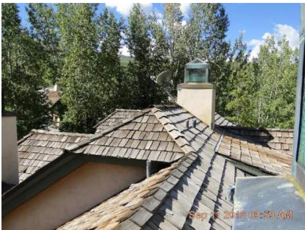
Top of roof from the east end facing west.
