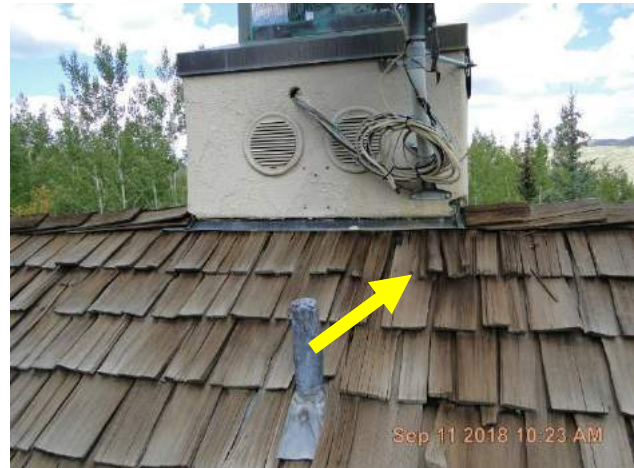
Copper transition metal and W-Valley metal at back, rear dormer
