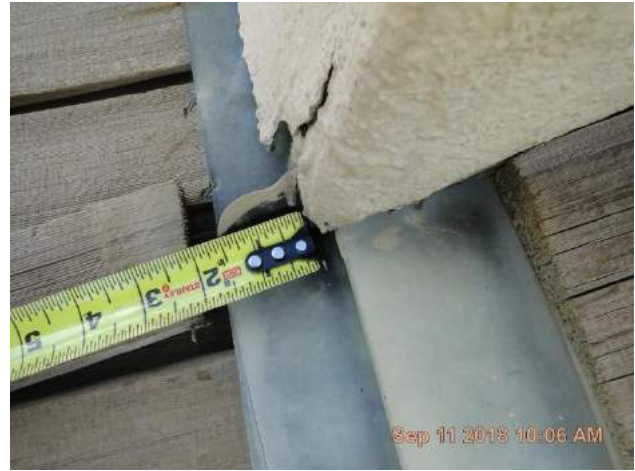
Close up of side wall to head wall flashing detail at chimney shows 1-1/4" high x 1-1/2" long kick-out flashing
