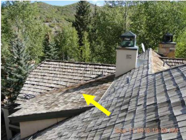
There are several lower slope dormer shed roofs that register at a roof slope of 2.5 to 3 requiring double felt.
