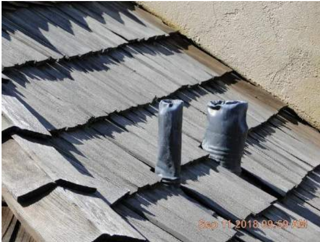
Lead pipe vent flashings (pipe jacks).
