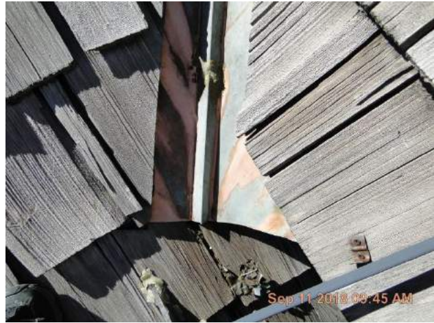
End of copper valley at side wall.
