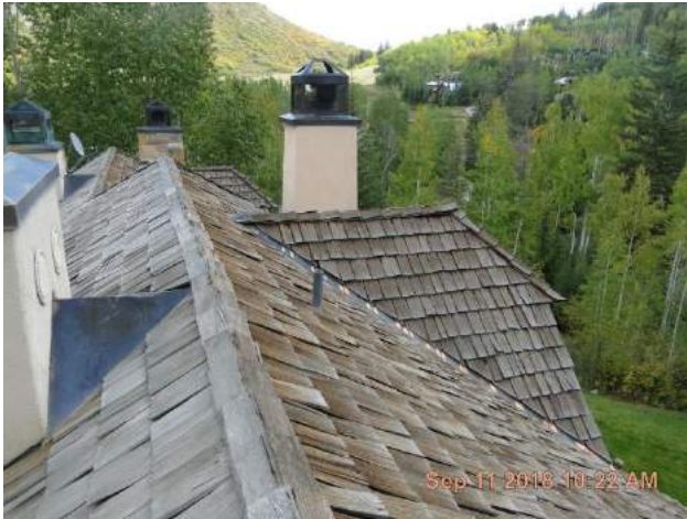
Top of roof from the west end facing northeast.
