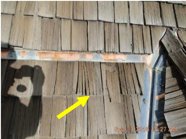
Back (south) elevation shows a considerable number of split shingles.
