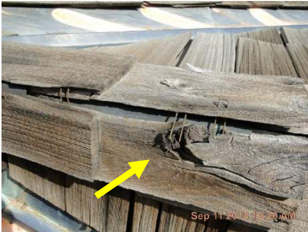
Badly split and rusted ridge shingle.
