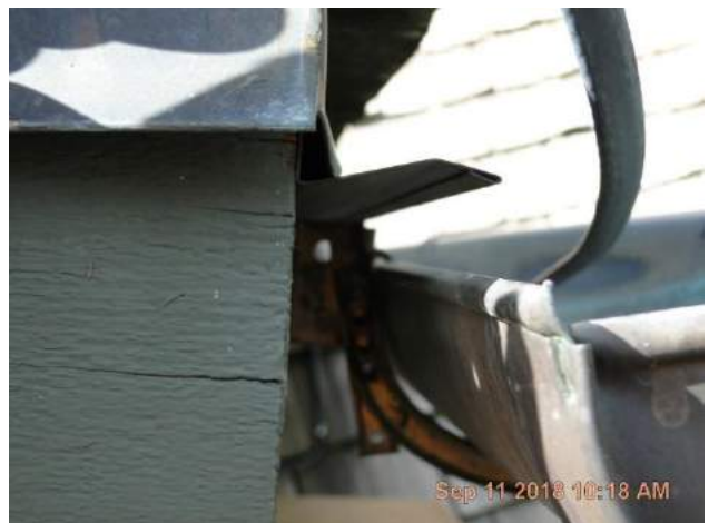
Close up of gable to eave transition shows close up of gutter and gutter attachment.
