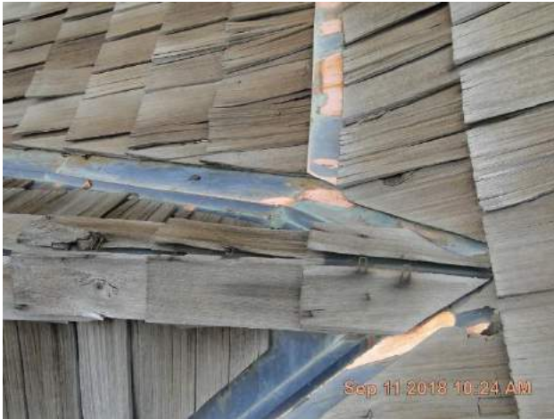
Ridge cap at back slope is split from the 2-inch staples rusting out. There is 10-inch copper step flashing installed under the wood shake at the ridge cap to protect the roof.
