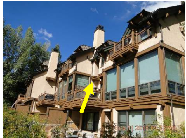
Back (south) elevation at right end.
