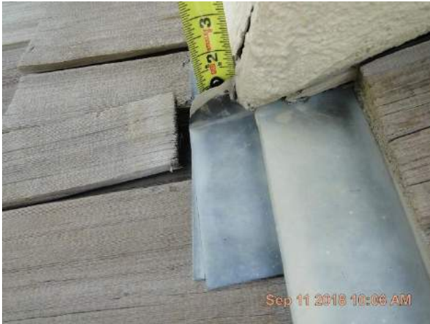
Close up of side wall to head wall flashing detail at chimney shows 1-1/4" high x 1-1/2" long kick-out flashing
