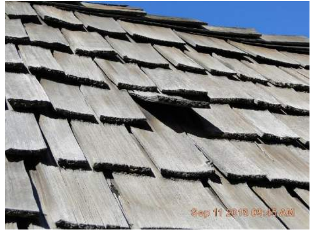
Curled shake shingle at front dormer is at higher risk to crack and separate from the roof.
