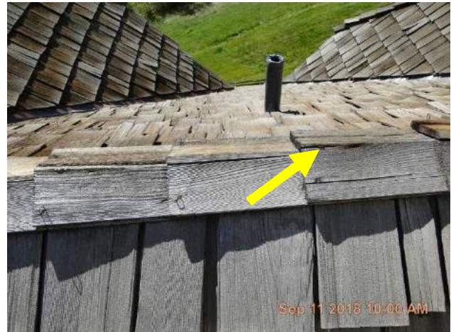
The ridge cap is a standard medium wood shake ridge cap that is staples together. These staples rust over time causing the ridge cap to separate and split.
