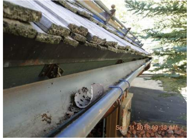
Front eave over garage shows drip edge and half Round copper gutter.
