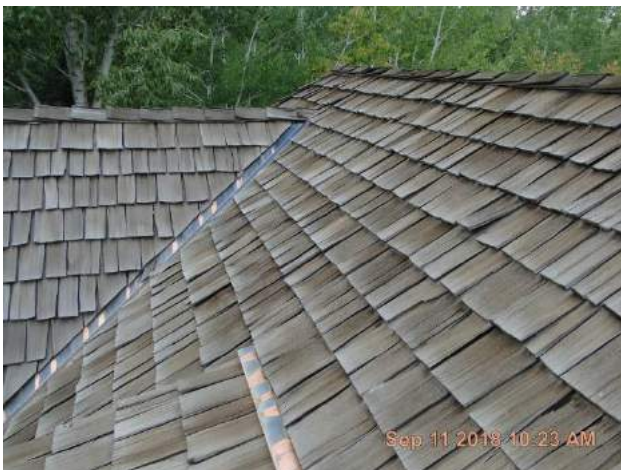
Back roof slope.
