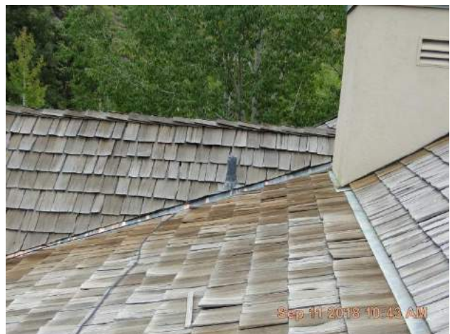
Low slope roof at the back elevation is badly worn.
