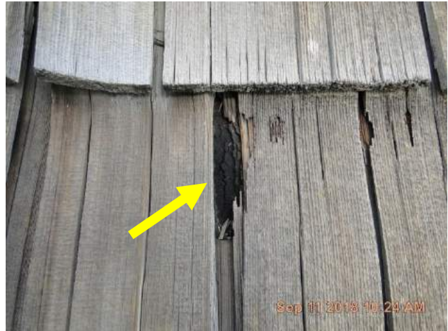
Close up of wood shake shingles with holes worn through them shows the top layer of felt has also been worn through leaving the bottom layer of ice & water shield remaining to protect the roof deck and interior.
