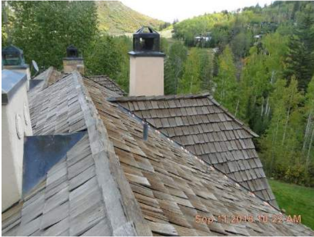
Top of roof toward the middle facing south
