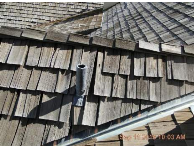
Left (west) side of front dormer shows some split shingles and others that are curled up do to the uneven Drying of wood shake that occurs over solid sheathing.
