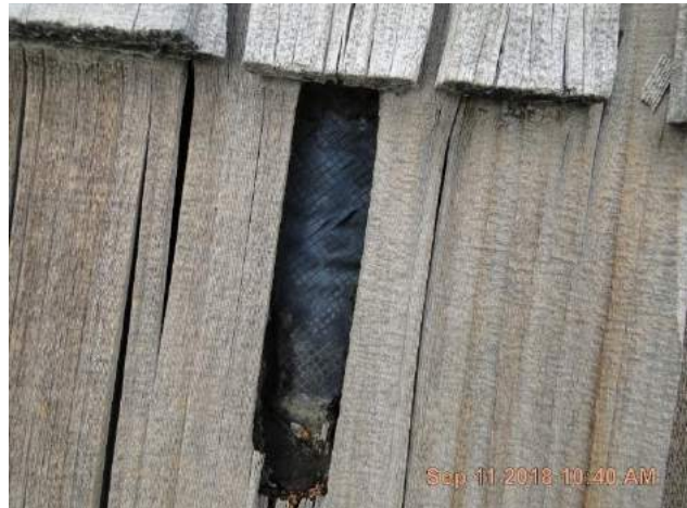
Large hole in shingles shows exposed ice and water shield below interlacing felt.
