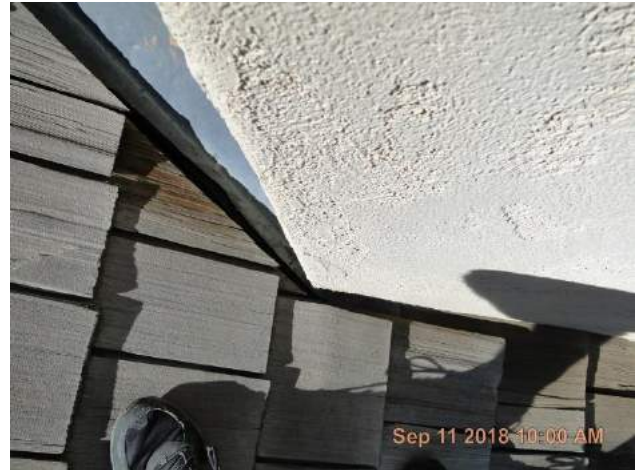
Closeup of chimney at cricket valley to side wall.
