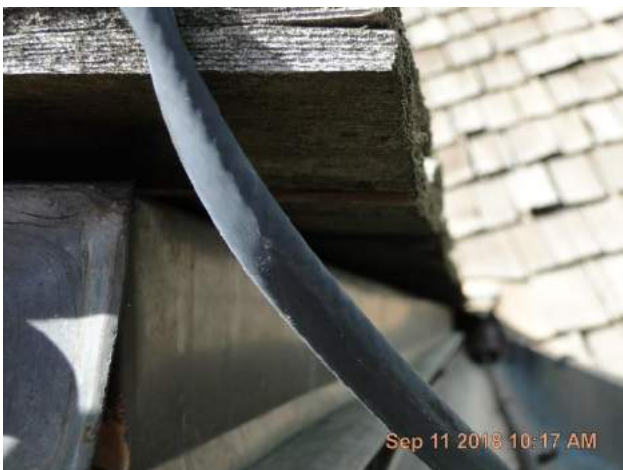
Close up of heat tape / cable also shows a gap at the rake metal to drip edge transition.
