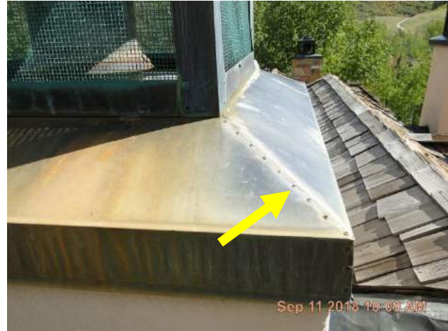
Copper chimney chase with screened cage around chimney flue. Chase is riveted and soldered together.
