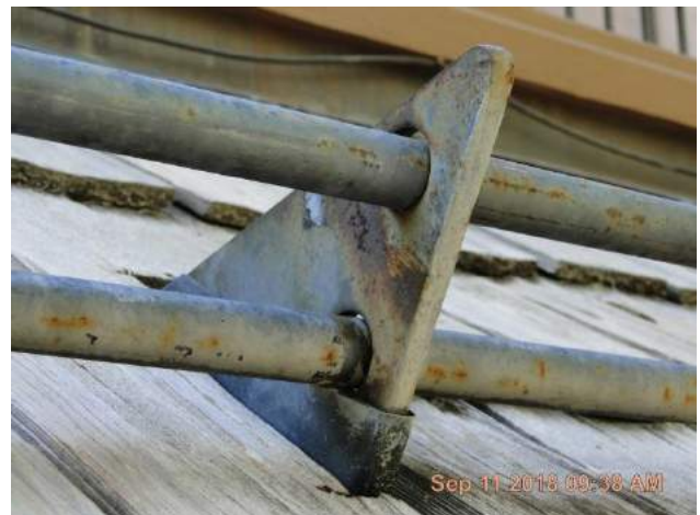
Closeup of snow fence bracket.
