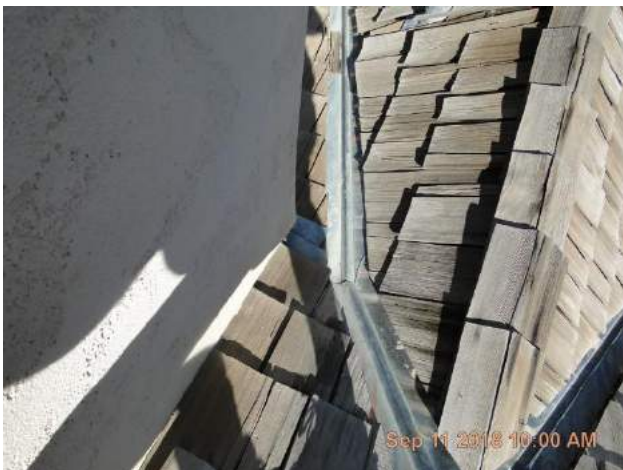
Copper valley at chimney side wall.
