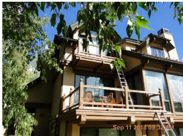
Back (south) elevation at left end.
