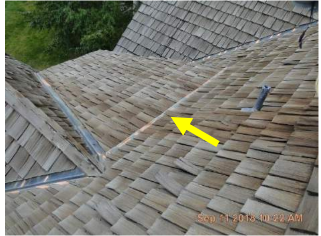
Transition from steep to lower slope roof at the back (south) elevation.
