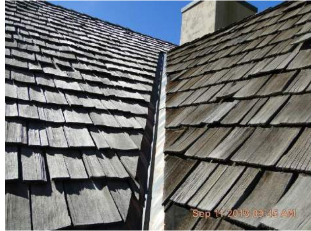
Front roof slope at steep 10/12 front dormer.
