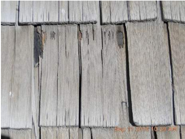
Close up of wood shake shingles with holes worn through them shows the top layer of felt has also been worn through leaving the bottom layer of ice & water shield remaining to protect the roof deck and interior.
