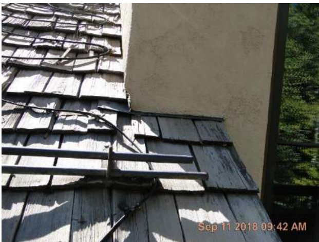
Front roof head and side wall at left of deck.
