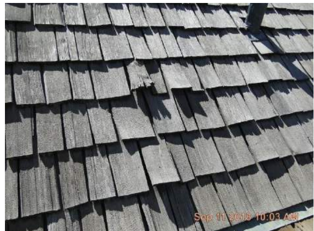
Left (west) side of front dormer shows some split shingles and others that are curled up do to the uneven Drying of wood shake that occurs over solid sheathing.
