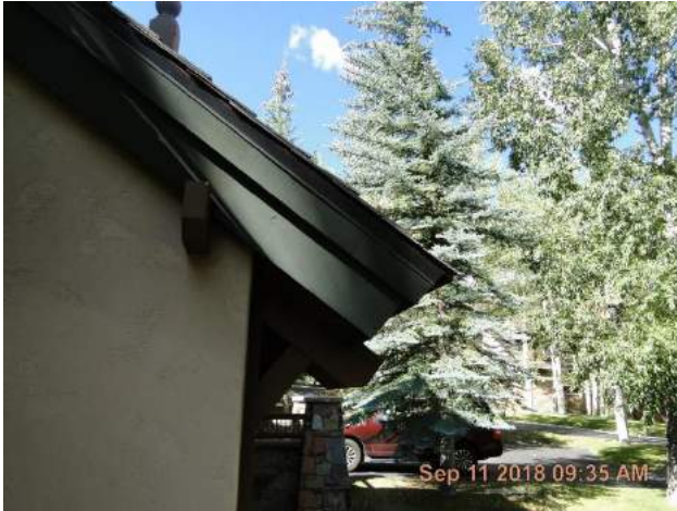
Rake edge at front left gable.
